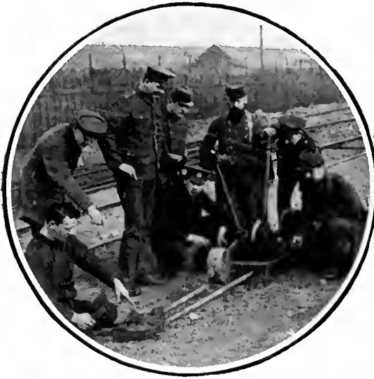
Repairing a railway point.
